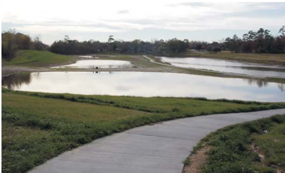
Construction of the Freshwater Tidal Marsh was completed in January 2006. The tidal marsh is just one of the many projects the Harris County Flood Control District is undertaking to reduce flood damages while incorporating community and natural values along Brays Bayou.
