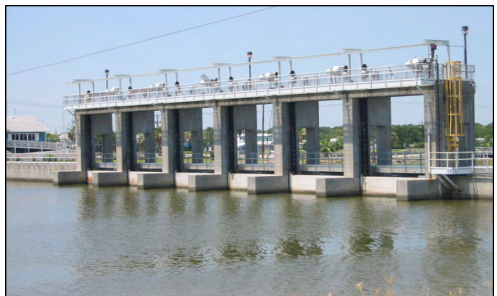
Gated Structure in Clear Lake City HCFCD Unit A200-00-00
