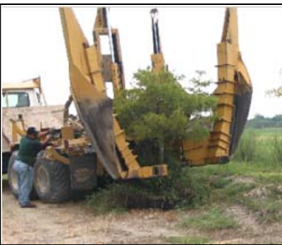
Tree Spading in HCFCD Basin C500-01-00.
