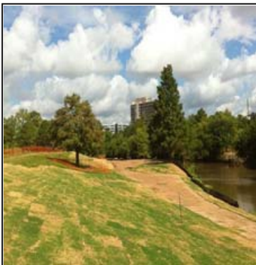
Buffalo Bayou Pilot Project (HCFCD W100-00-00).
