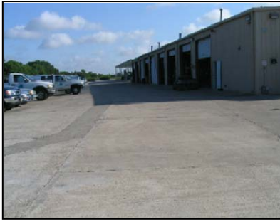
South Service Center Mechanics Shop.
