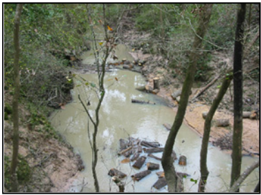
Desnag project along Unit L100-00-00 (Little Cypress Creek).
