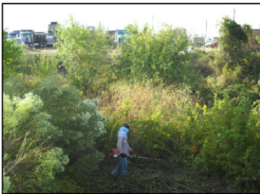
Selective clearing in progress downstream of Fairbanks N. Houston.
