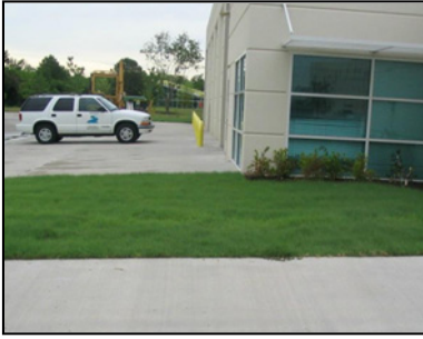
North Service Center Fleet Maintenance Shop Area.
