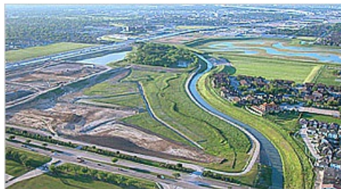
The Arthur Storey Park Stormwater Detention Basin, at Brays Bayou near W. Sam Houston Tollway, is a massive flood damage reduction complex with park amenities.
