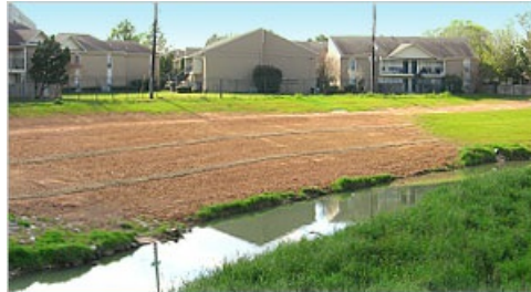
Portion of the completed Greens Bayou slope erosion repair project.
