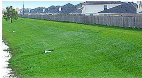
Newly restored bank of a tributary of Dinner Creek, located in the Addicks Reservoir watershed.
