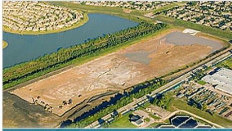
Old Westheimer Road Stormwater Detention Basin. Under construction.
