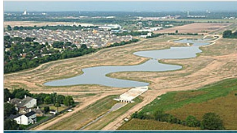
Mason Creek Extension and Detention Basin, Near Completion
