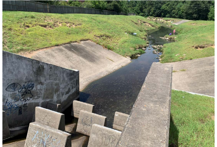
Drop structure at Taylor Gully
