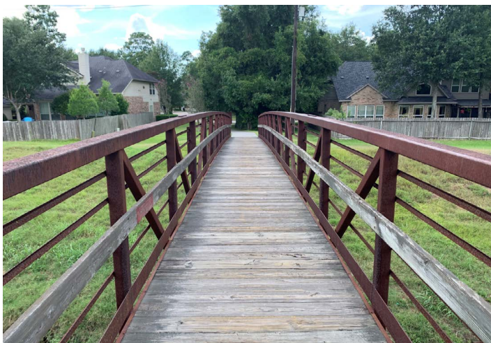
Pedestrian Bridge Over Taylor Gully
